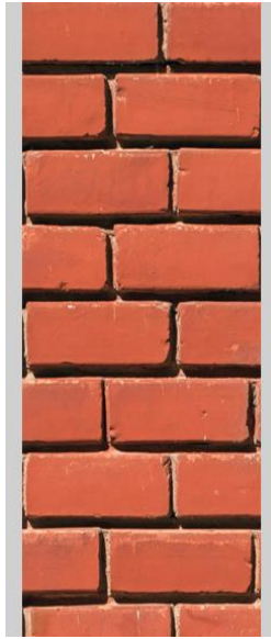
Hollow Brick Wall
