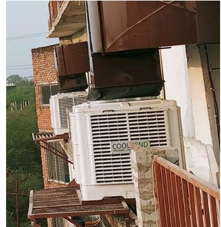
Hostel, Lucknow, India
